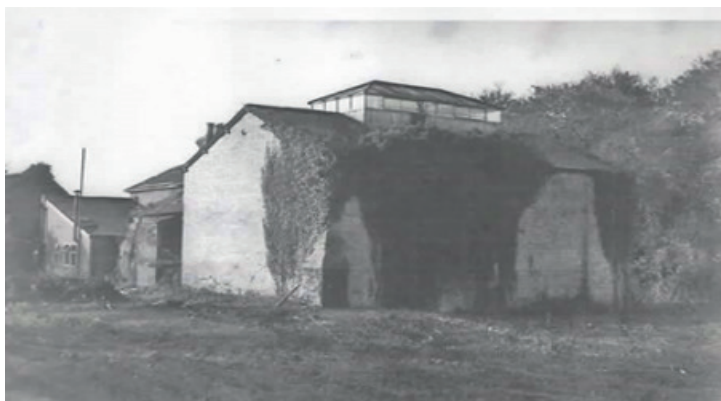
The retort house before it was demolished
