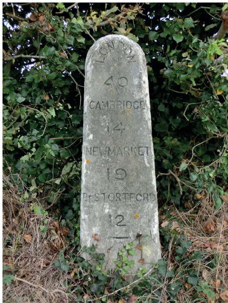
Incised benchmark on milestone 40 south of Littlebury.
