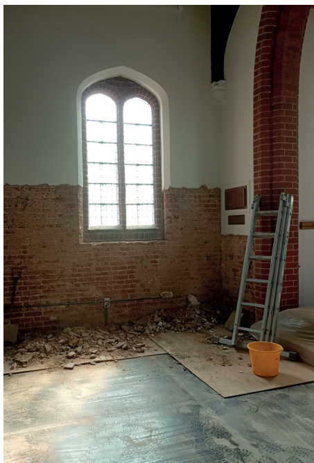
The Brick Work
