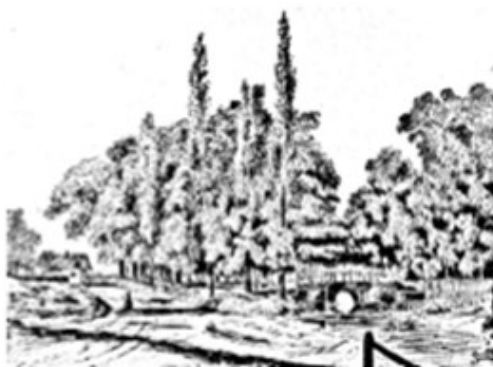
Wyddial Road and Little Court Bridge 1839
